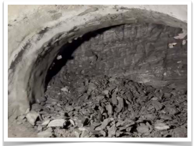
Tunnel After Blasting and Scaling
